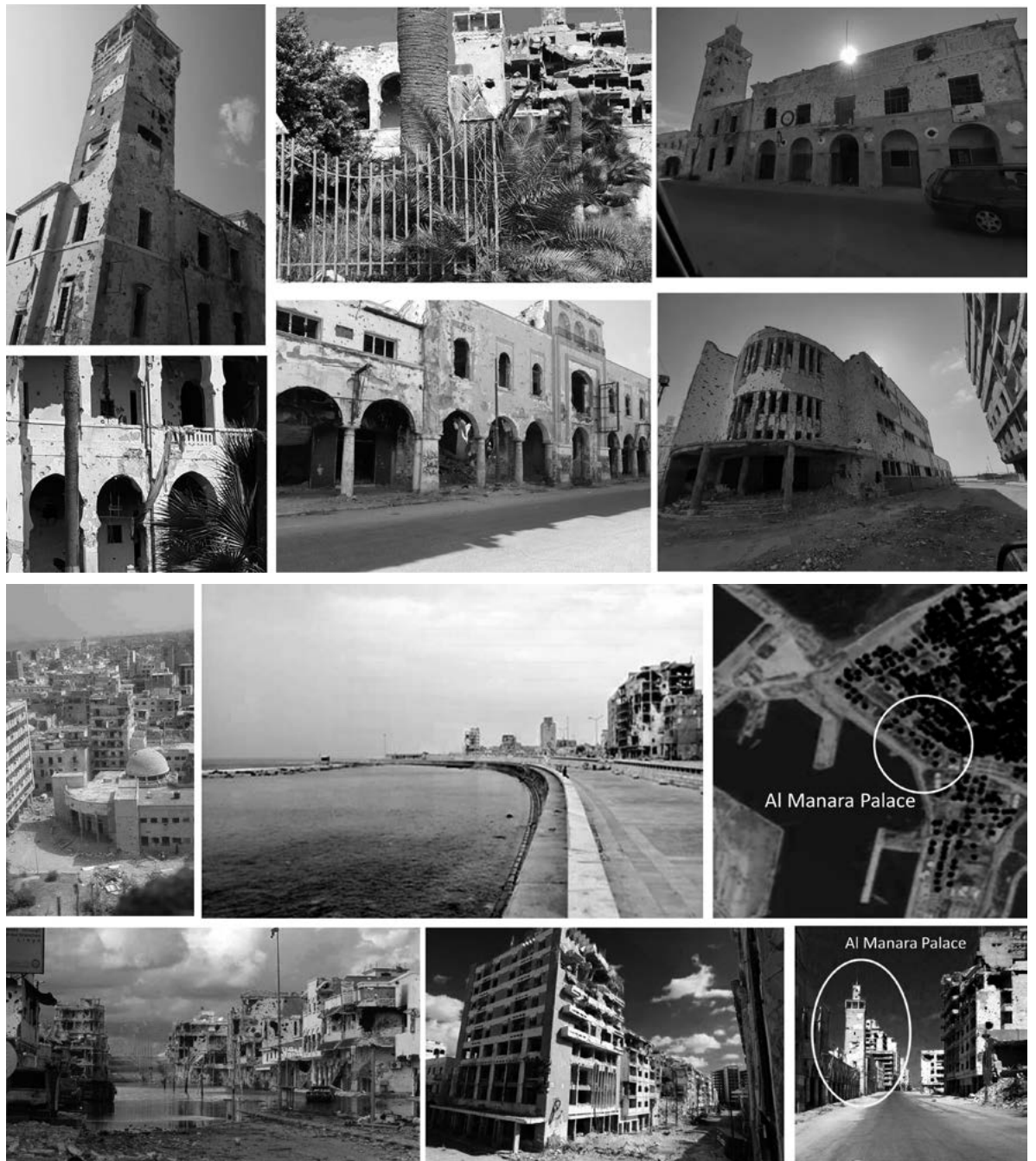
Figure 4: Damage assessment to the building (first 6 images) and its surrounding area (last 6 images).
