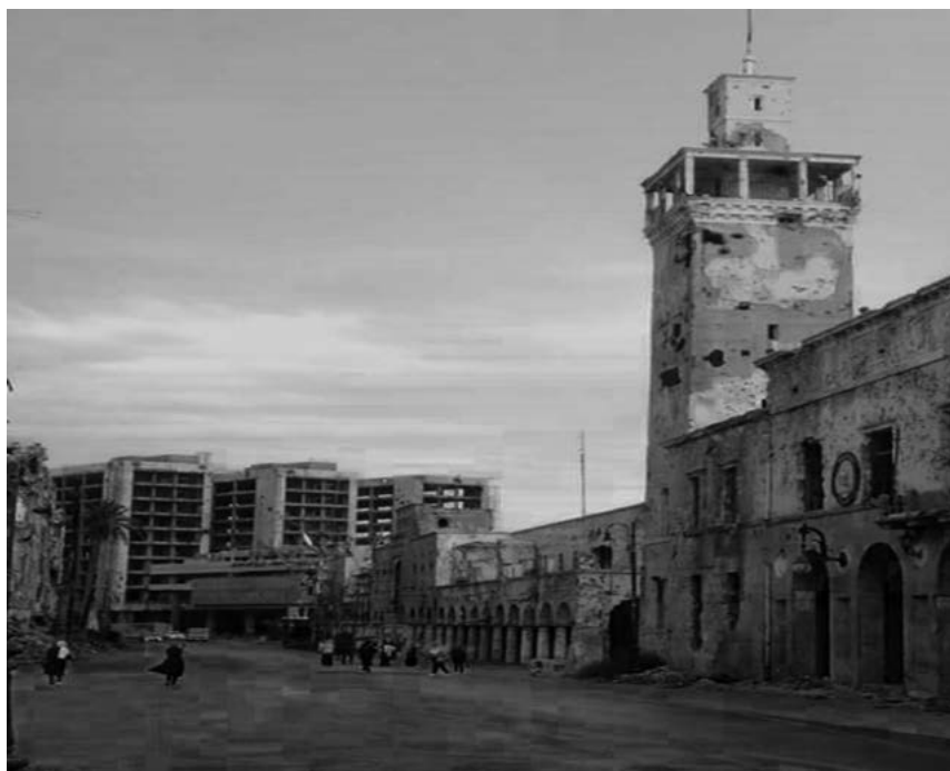
▲ Figure 1: The damaged Al-Manara Palace in Benghazi. Source: EUC, Benghazi, 2019.
