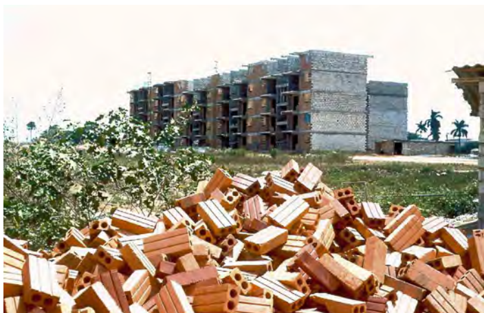
Standard mass housing system being built on virgin land.
