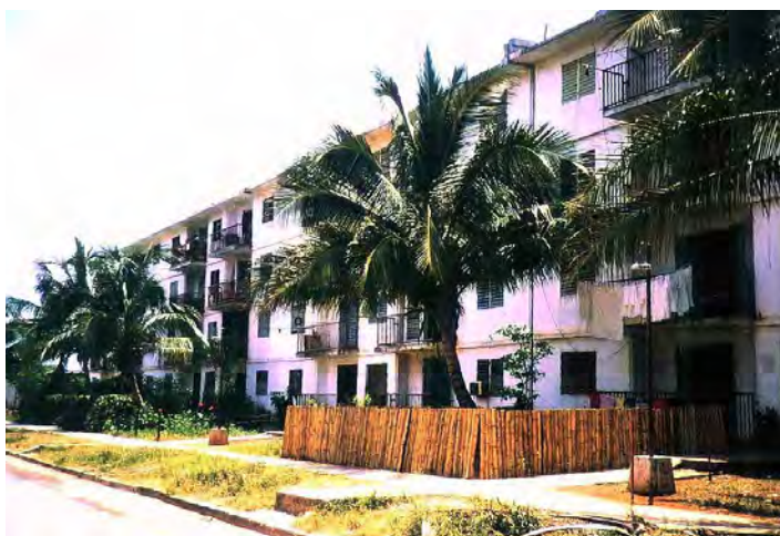
Standard mass housing system being built on virgin land.
