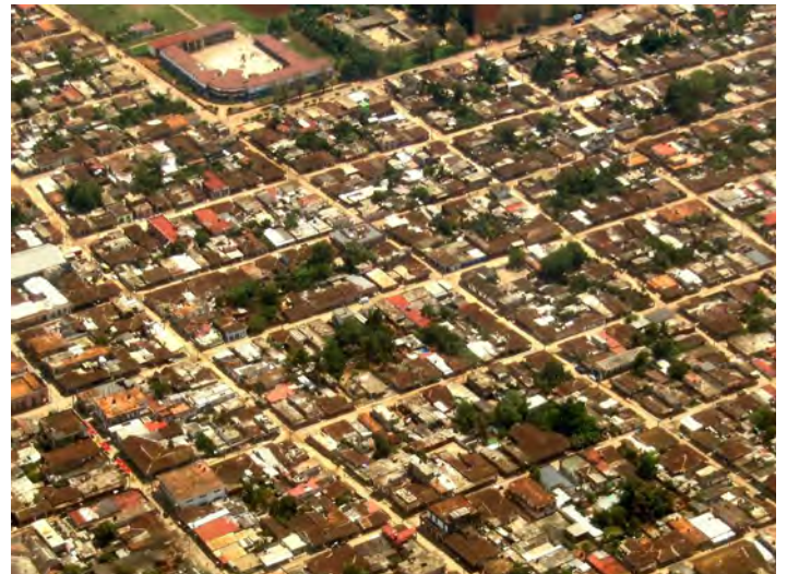
Small town in Havana province. One-storey development on a grid-iron street pattern
