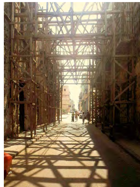
Securing existing facades before reconstruction in Old Havana
