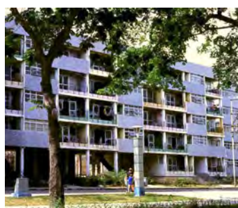
State built industrialized housing usually is limited to a few standard plans and at least partially prefabricated. Here: in Central Havana.
