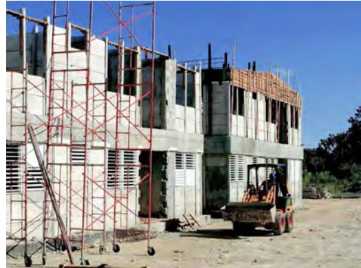
Emergency housing being built with Sandino system in Havana Marionao 2013
