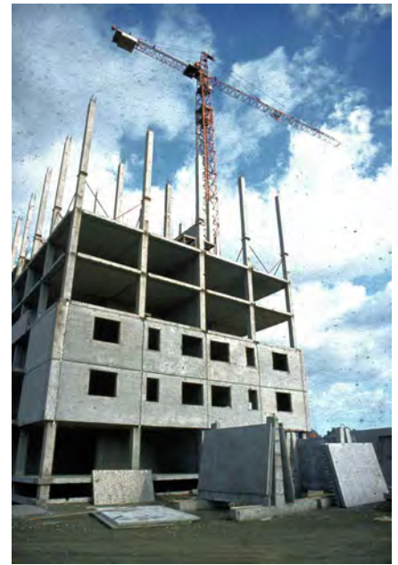
In central and Western Cuba, the Yugoslavia IMS column-based construction system was used and allowed high-rise building of up to 11 floors.
