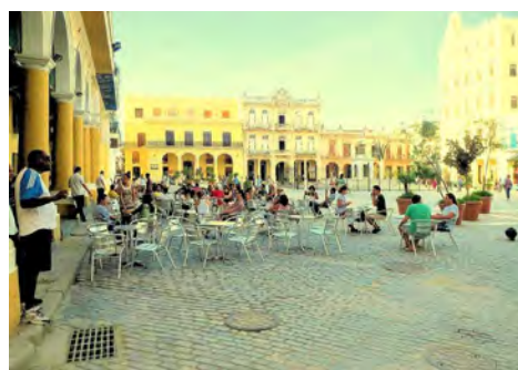
Almost all buildings around the Plaza Vieja were dilapidated and have been restored offering apartments for the displaced families
