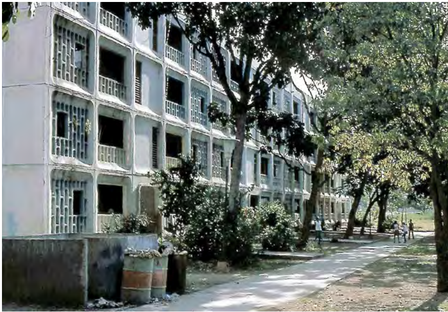
Imported prefabrication system from the Soviet Union with reinforced façade panels to increase Earth-quake resistance, used in the extreme Eastern parts of Cuba – locally nicknamed ‘el televisor’. Because of the tropical climate, the panels were perforated with holes to allow ventilation.
