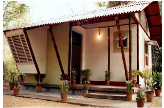
House built of Bamboo, developed in the University of Santiago de Cuba. (Photo: Juan Manuel Pascual Menendez, CASAS, Universidad Santiago de Cuba)
