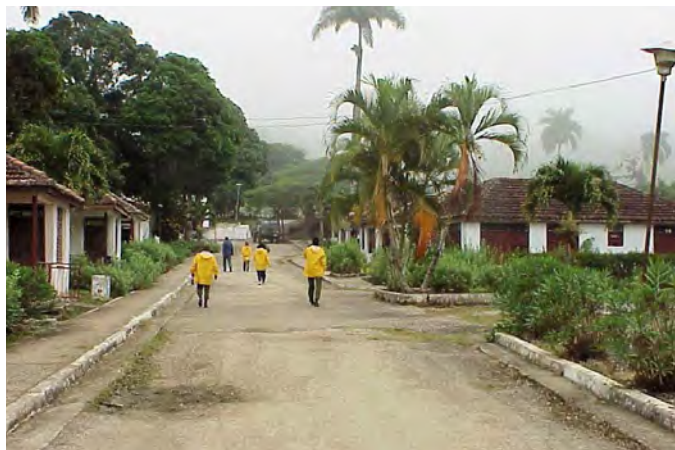
New village built as part of the Plan Turquino in Eastern Cuba (Photo provided by Milagros López)
