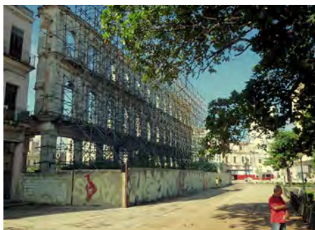
Reconstruction of historic structure in Old Havana
