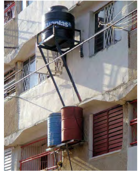
Water supply is provided to all households, but the service can be irregular. Therefore, many residents install a personal water tank to assure uninterrupted availability.
