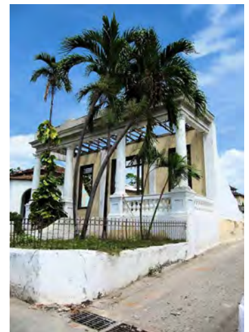
Damages of Hurricane Sandy in Santiago de Cuba, 2012
