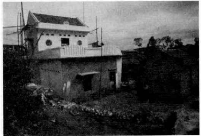
CURRENT CONSTRUCTION IN VIETNAM. NOTE THE SIMPLE KITCHEN BUILDING ON THE RIGHT
