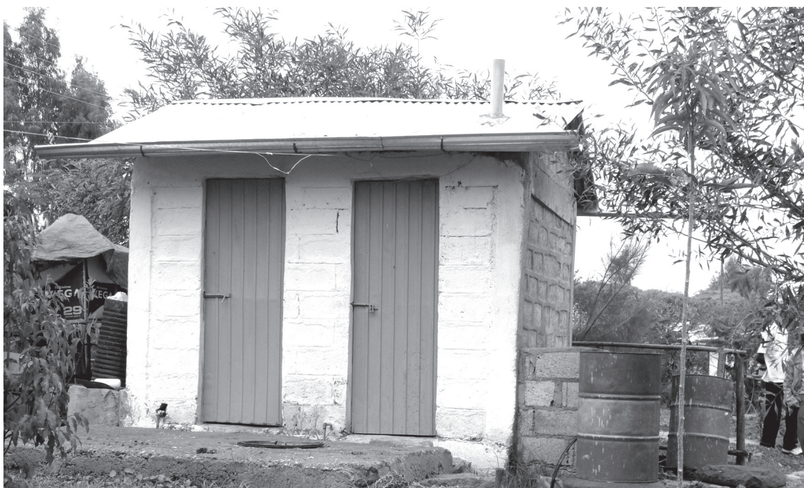
◀ fig 2: Biogas latrine operated by the youth group
