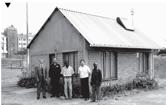
fig 3: Low cost energy house with solar thermal collector on the roof on the campus of the Witwatersrand University in Joburg
