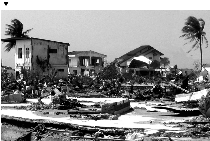
fig 1: Destructions in a residential area in Banda Aceh
