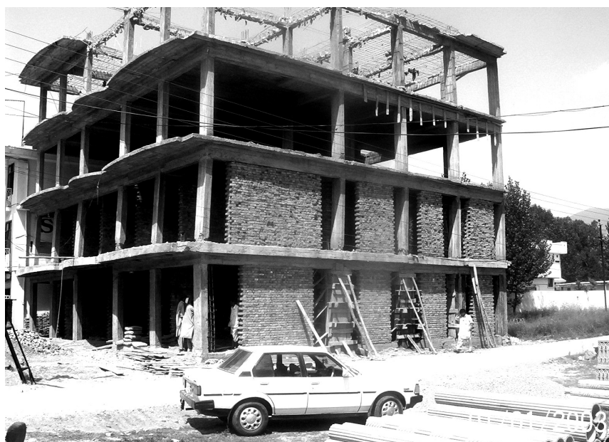
fig 2: Repair (continued construction) of an unsafe building in Abbotabad, Pakistan, that was damaged by the October 8, 2006 earthquake
