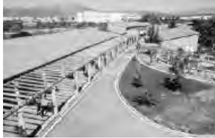
OLBIA SOCIAL CENTRE OF AKDEMIZ UNIVERSITY CAMPUS, ANTALYA, TURKEY. A SERIES OF BUILDINGS FOR STUDENTS AND TEACHERS, OFFERING ALSO SPACES FOR THE PUBLIC. ARCHITECT: CENGIZ BAKTAS
