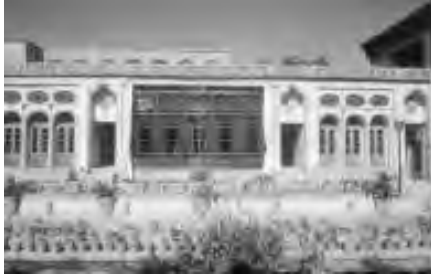
NEW LIFE FOR OLD STRUCTURES PROGRAMME AT VARIOUS LOCATIONS IN IRAN. A'LAM VA'EZ RESIDENCE IN ISFAHAN
