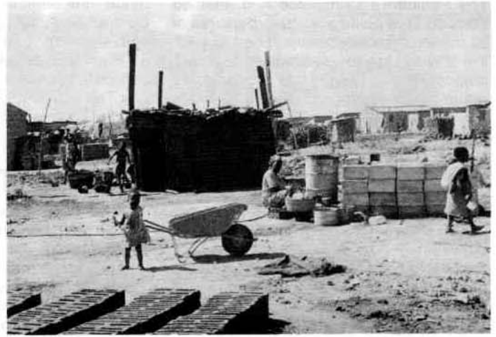
Building a house
