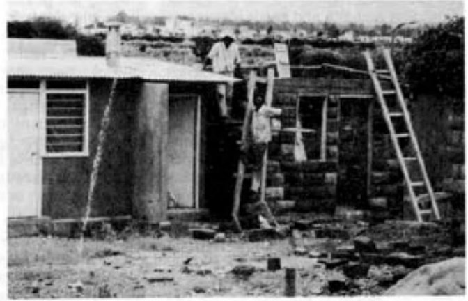
Dandora: Construction work in progress, 1977. (Photo: H. Schmetzer)
