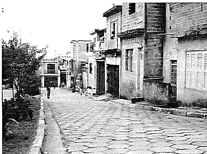
Fig. 2: Favela upgrading with street paving and infrastructure provision: the neighbourhood Vila Nova (1995)
