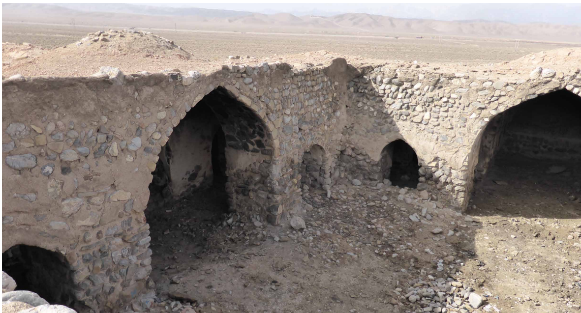
► Figure 3: The courtyard of the caravan serai. Photo: Renate Bornberg
