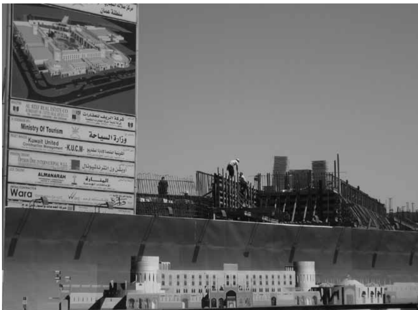
▼ Figure 4: Salalah Gardens Mall under construction (Source: Steffen Wippel 2010)
