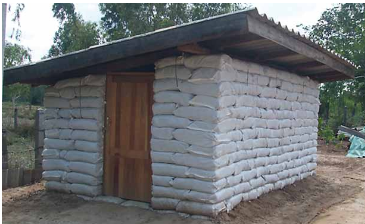
▼ Figure 7 and 8: Shelter during construction process. Photos by Chankamol Kumjuang
