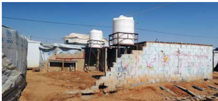
▲ Figure 3: Sanitary facilities in Zaatari Camp, Jordan. Photo: Ayham Dalal, 2014
