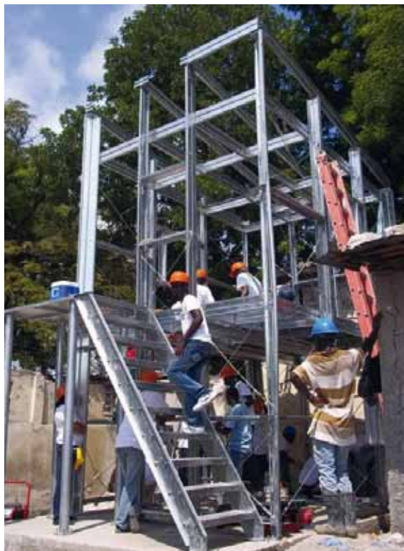
Figure 18: KATYE shelter under construction – steel structure. Photo by Kendra Helmer, USAID
