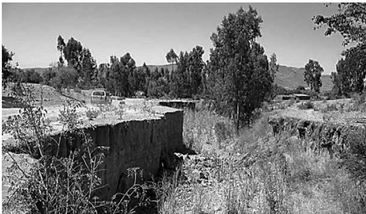
Figure 8: The gully formed after a street washed away. Photo: J. Schoeneberger
