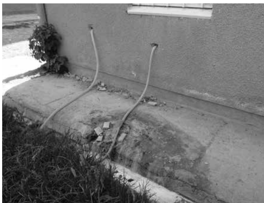
▼ Figure 6: Wastewater from a hairdresser led into the rainwater drainage, Bole Gerji V. Source: M. Wiebusch 2009
