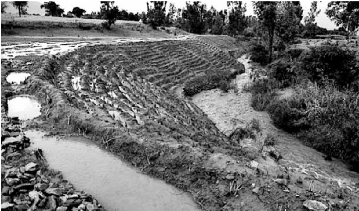
◀ Figure 6: Small terraces built for planting bushes to stabilise a slope. Photo: J. Schoeneberger
