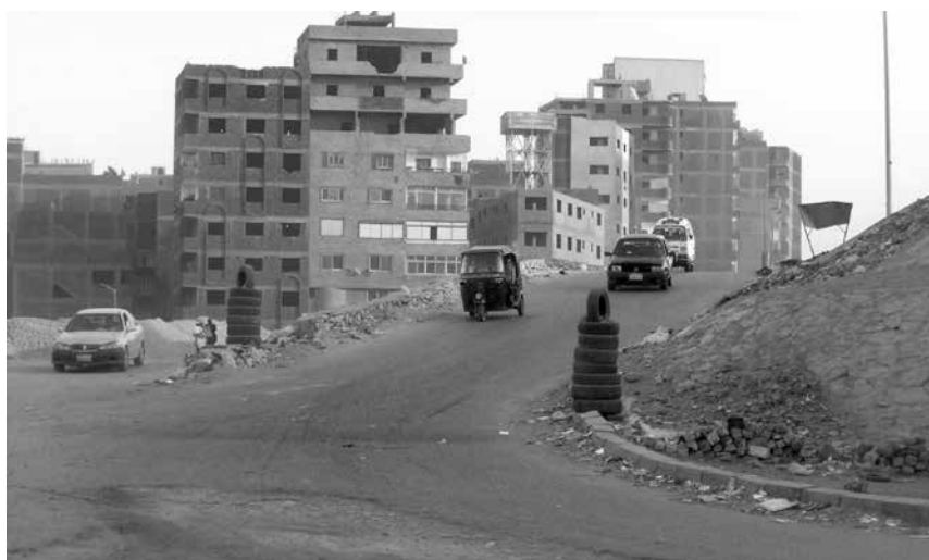
▲ Figure 11: Ring Road ramps after construction. Source: Abbas (2013)
