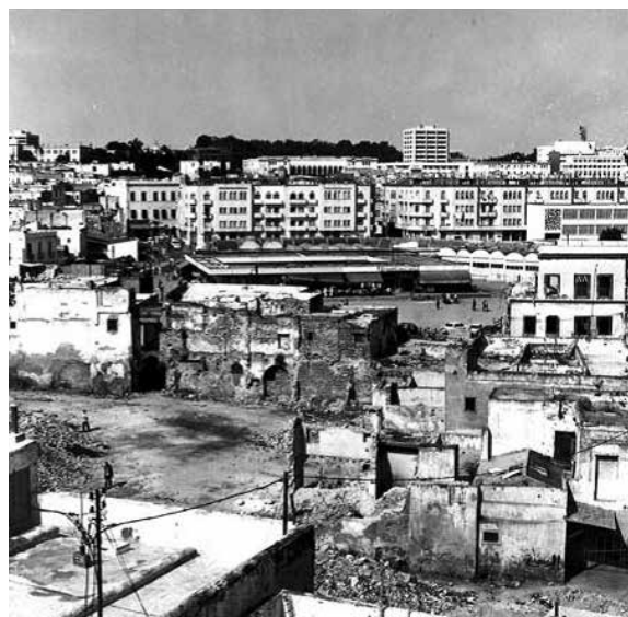
Figure 2: View of El Hafsia quarter, Tunis, prior to the rehabilitation. Source: AKAAs (1995: 46), available at: http://www.akdn.org/sites/akdn/files/media/documents/AKAA_press_kits/1995/Hafsia_Quarter_II.pdf [last accessed Feb. 5, 2018]
