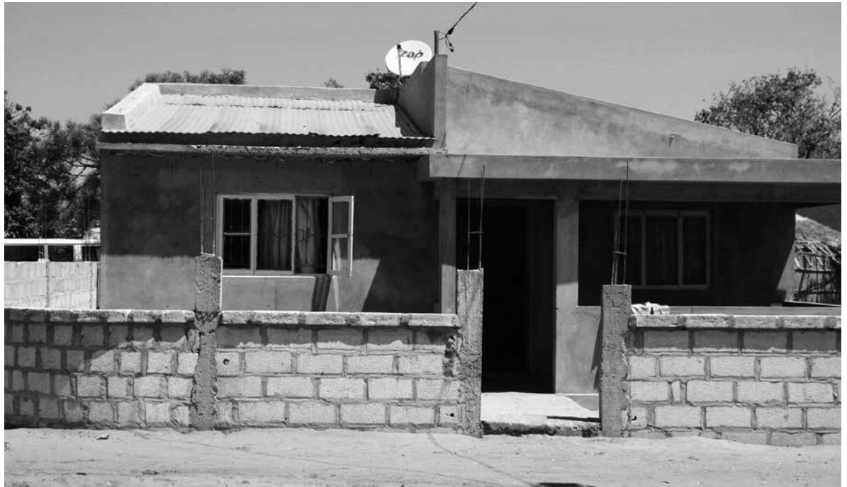
Figure 1: House under construction in Costa do Sol, Maputo. Photo: A. Mazzolini 2015
