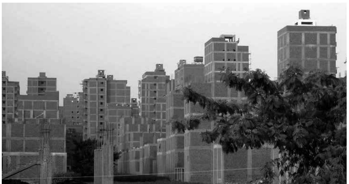
▶▶ Figure 5a and 5b: Speculative high-rise towers in well located and accessible parts of the informal area Bulaq-al-Dakrur. Source: the author
