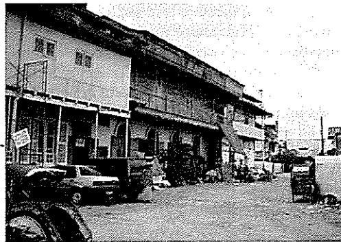
Fig. 6 / Neglected infrastructure in Jl. Kepodang / Photo: Marita Schnepf-Orth
