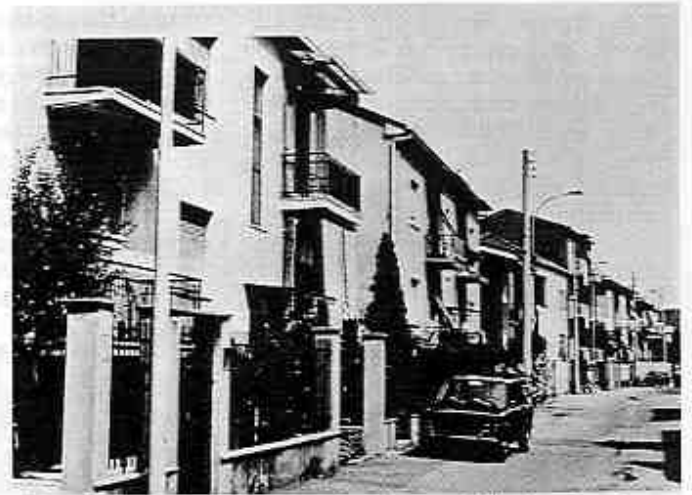
Fig. 7: Rome: Illegal apartment housing – middle class housing (source: exhibition on Rome: The Spontaneous Metropolis , 1983).
