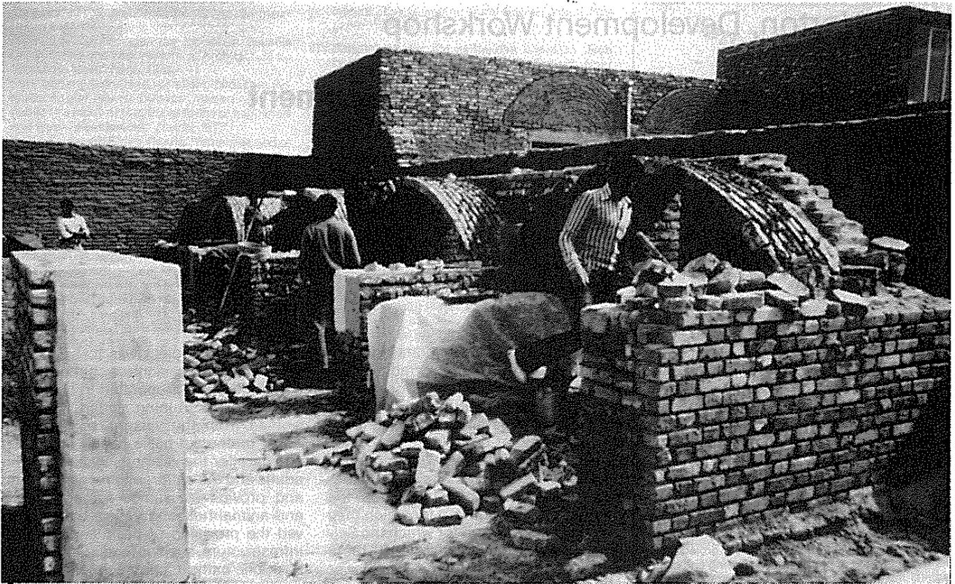
Fig. 2. Selseleh builders practising vault construction. In the foreground are wall and render test structures.
